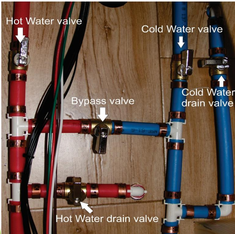
Valves are in winterizing mode after water was drained from the lines *(only needed if you're using RV antifreeze to winterize)*
