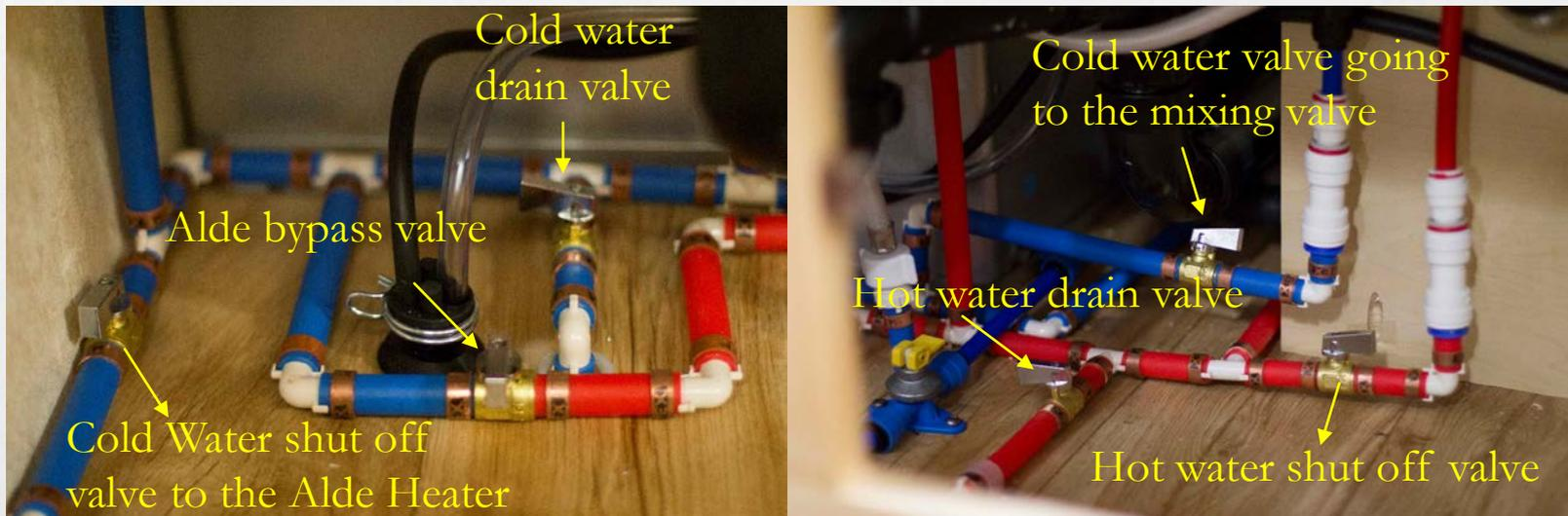
**Valves are in winterizing mode after water was drained from the lines.**
