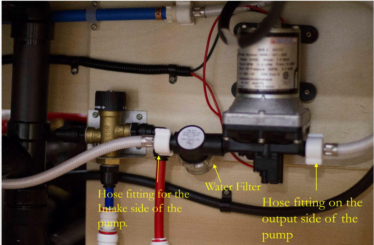
Hose fitting for the Intake side of the pump.
